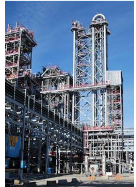
Borealis' polyethylene plant in Stenungsund.
